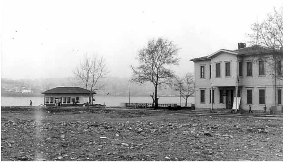
FENER ISKELESİ 1986 | VIEW OF FENER FERRY STATION AFTER LAND CLEARING
