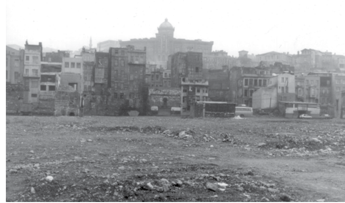
DEMOLITION OF INDUSTRY | 1986
